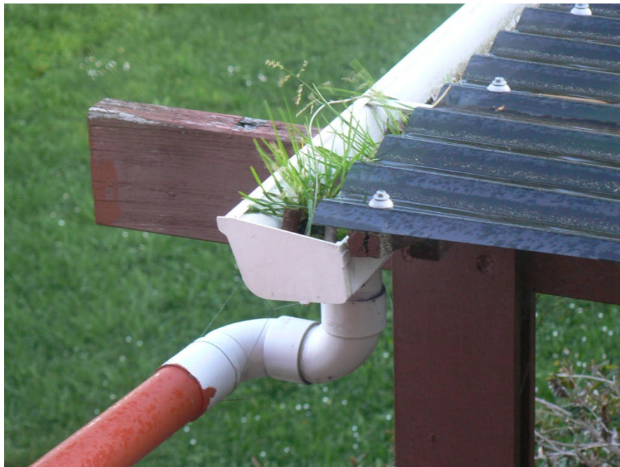
Gutter blocked at down pipe
