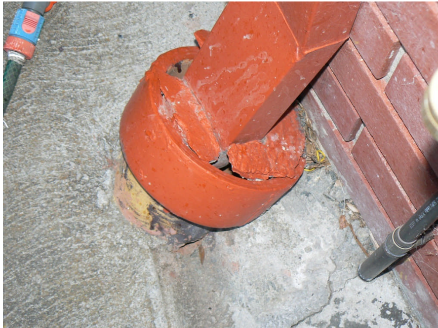
Stormwater pipe - cement cracked at earthenware pipe junction
